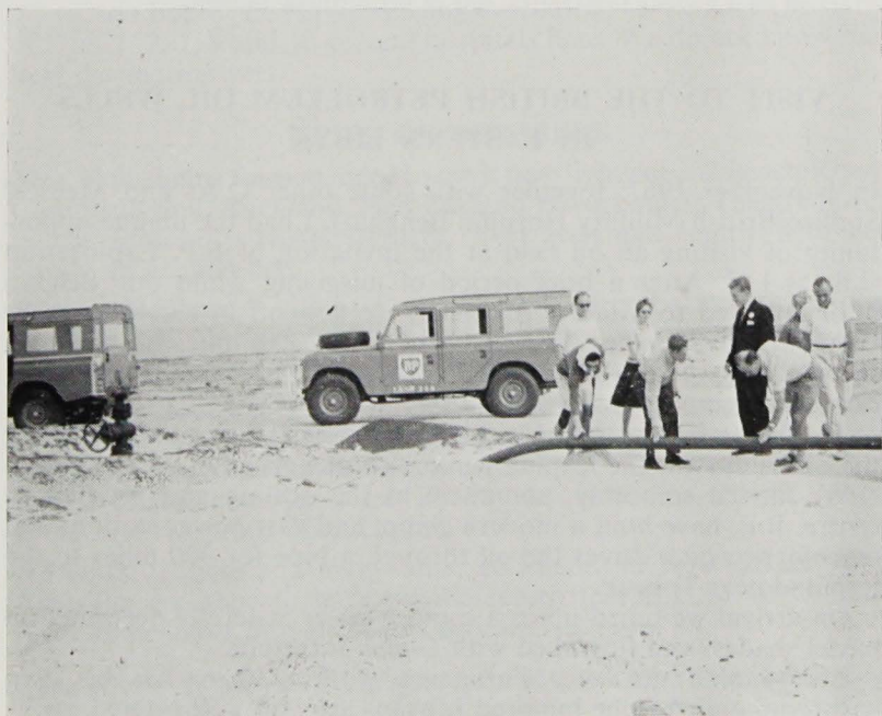
Feeling the hot pipes. The oil is at 200°F. and pumped from a mile below the surface.
