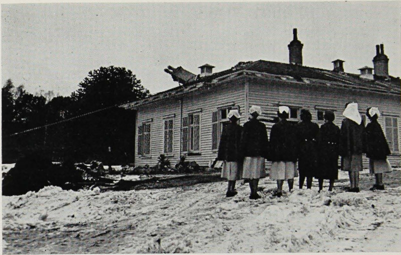
Demolition of the Royal Pavilion watched by members of the Staff of the Preliminary Training School.
