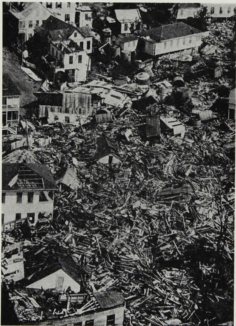
Three quarters of Belize's wooden homes were completely destroyed
